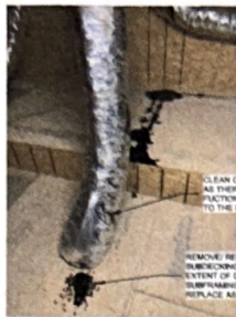
CONTRACTOR SHALL INVESTIGATE THE EXTENT OF DAMAGE ABOVE THE CEILING, PARTICULARLY WITH REGARD TO EXISTING CEILING FINISHES - I.E. SHALL CLEAN, REPAIR/REPLACE AS REQUIRED TO ENSURE TAN DAMAGE IS REMOVED.
